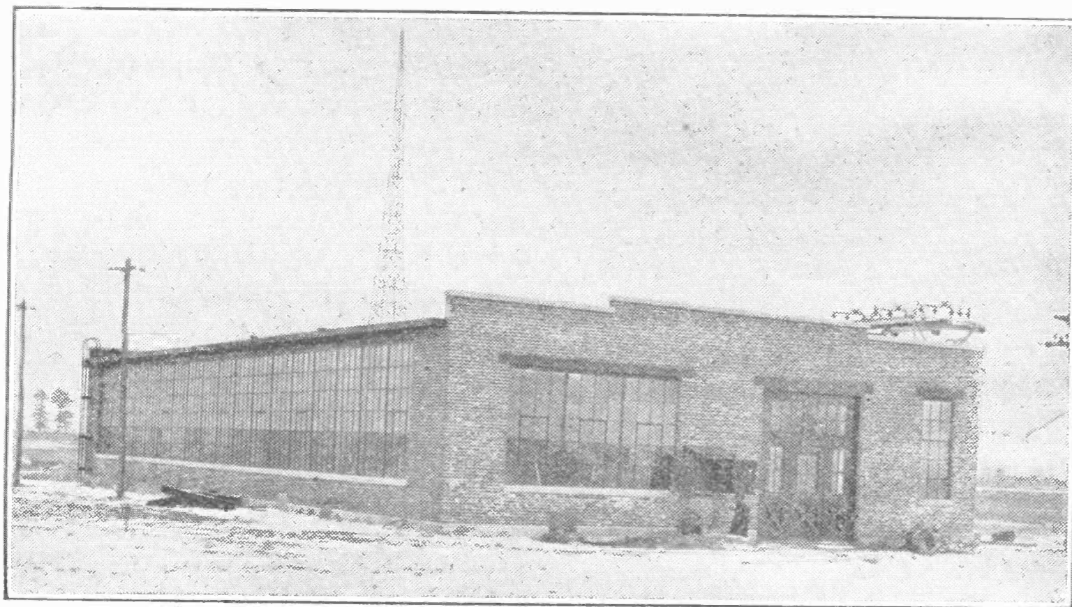
Fig. 4. Power House Will Take Up to 100,000 Watts
